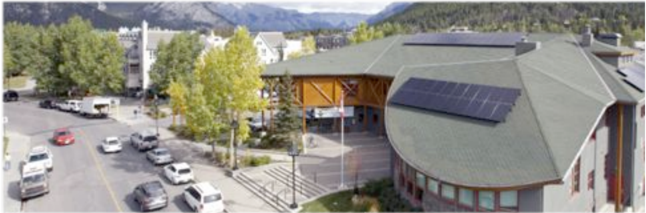
Figure 4. The Town of Banff installed solar panels on the roof of the Town Hall in 2013.
